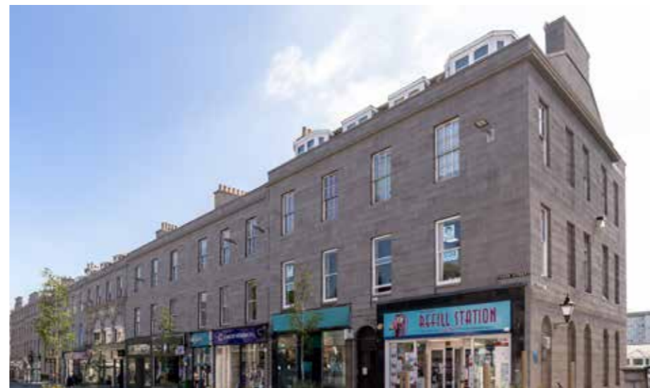
UNION STREET FACADE WORKS, SOURCE: ACC
