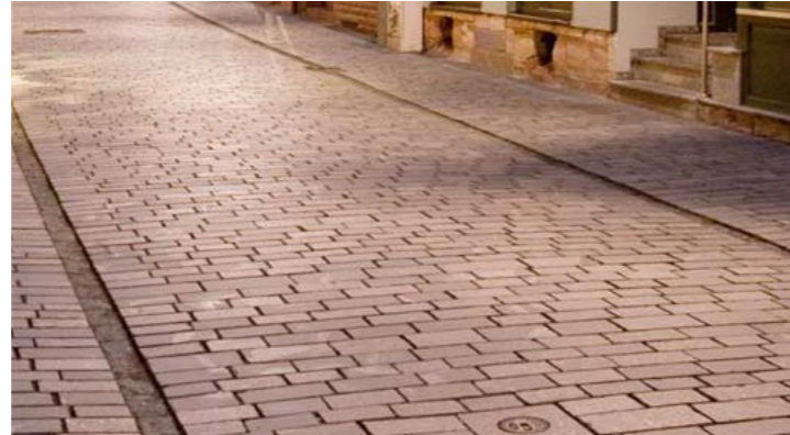
In ground lighting
